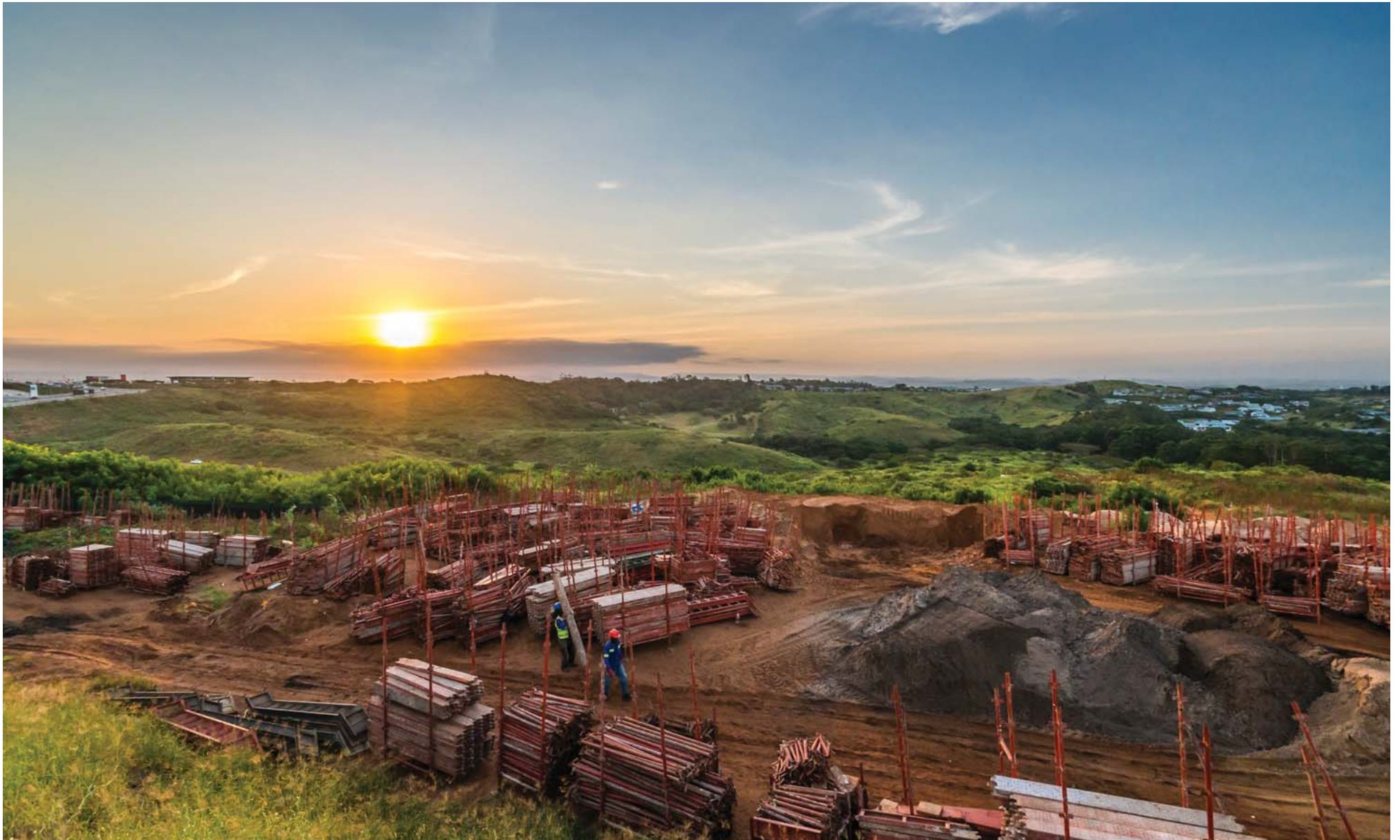
BALLITO HILLS CONSTRUCTION SITE
